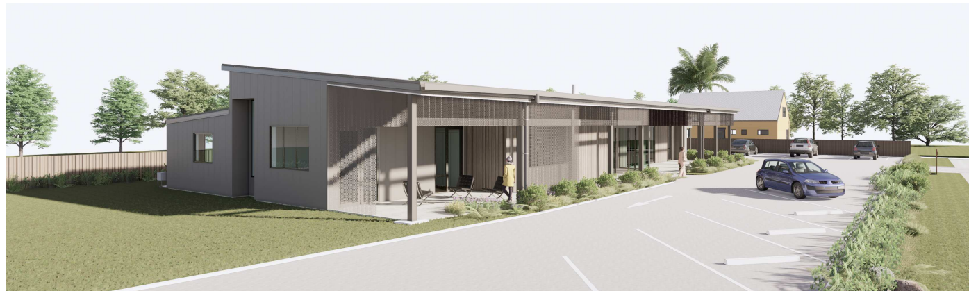
NORTH EAST VIEW - PHASE I
